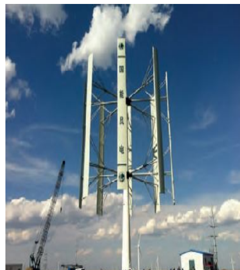
Fig. 2. Vertical-axis turbine
